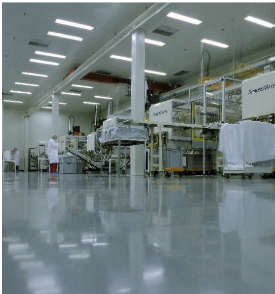
Figure 1 Cleanroom at MCAM Plastics NV
